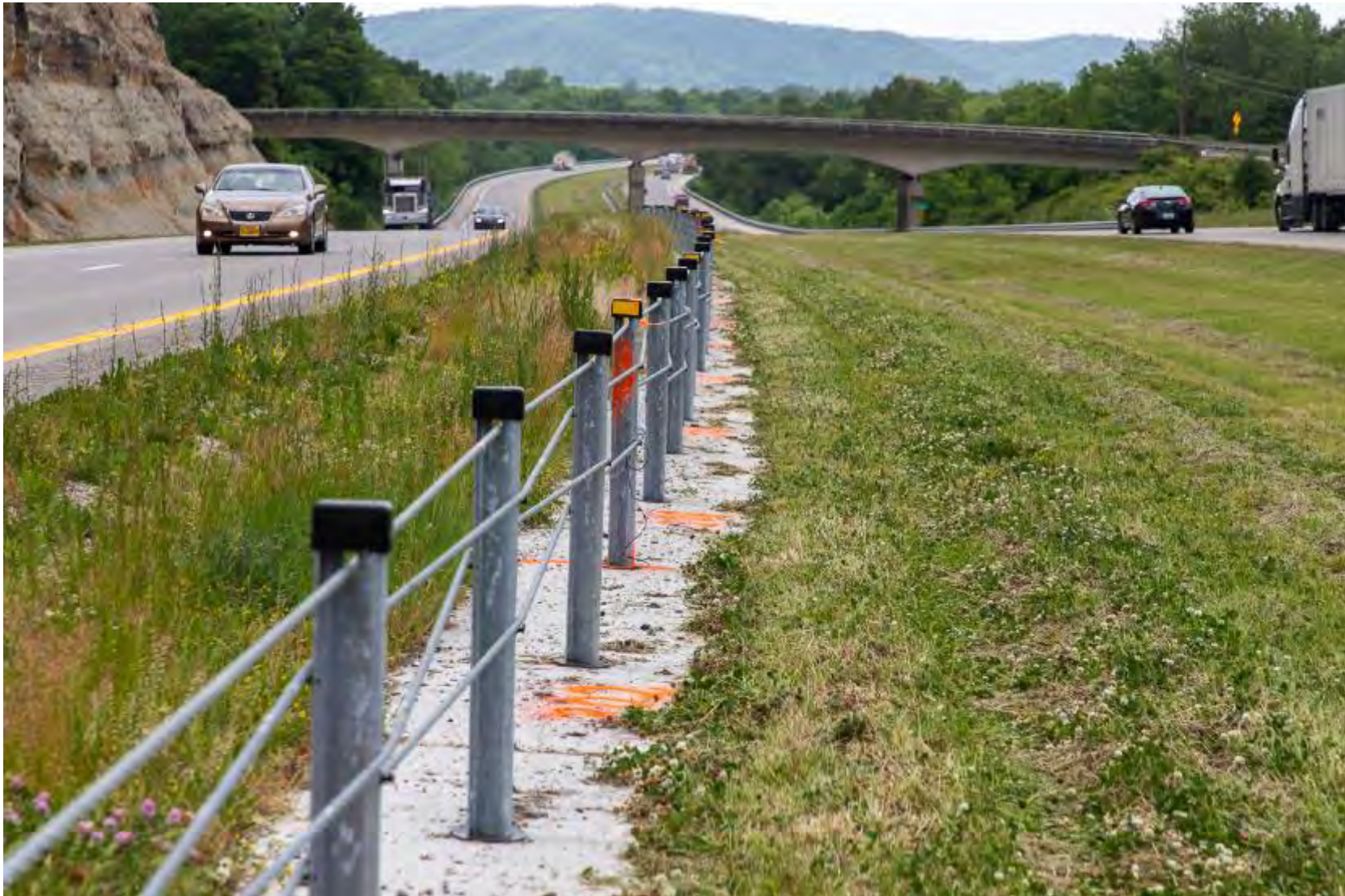
Figure 1: View of Plots in the Cable Barrier Trial near Morehead, KY on May 27, 2021 (Day of Treatment)
