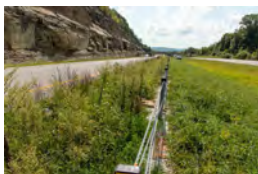
Figure 2: Overall view of cable barrier plots and surrounding area at time of Fall Application (September 14, 2021).
