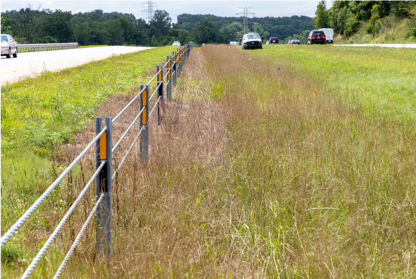
Figure 1: View of Plots in the Cable Barrier Trial on August 4, 2020 (63 Days After Treatment) Spray pattern observed on both sides of the cable barrier.
