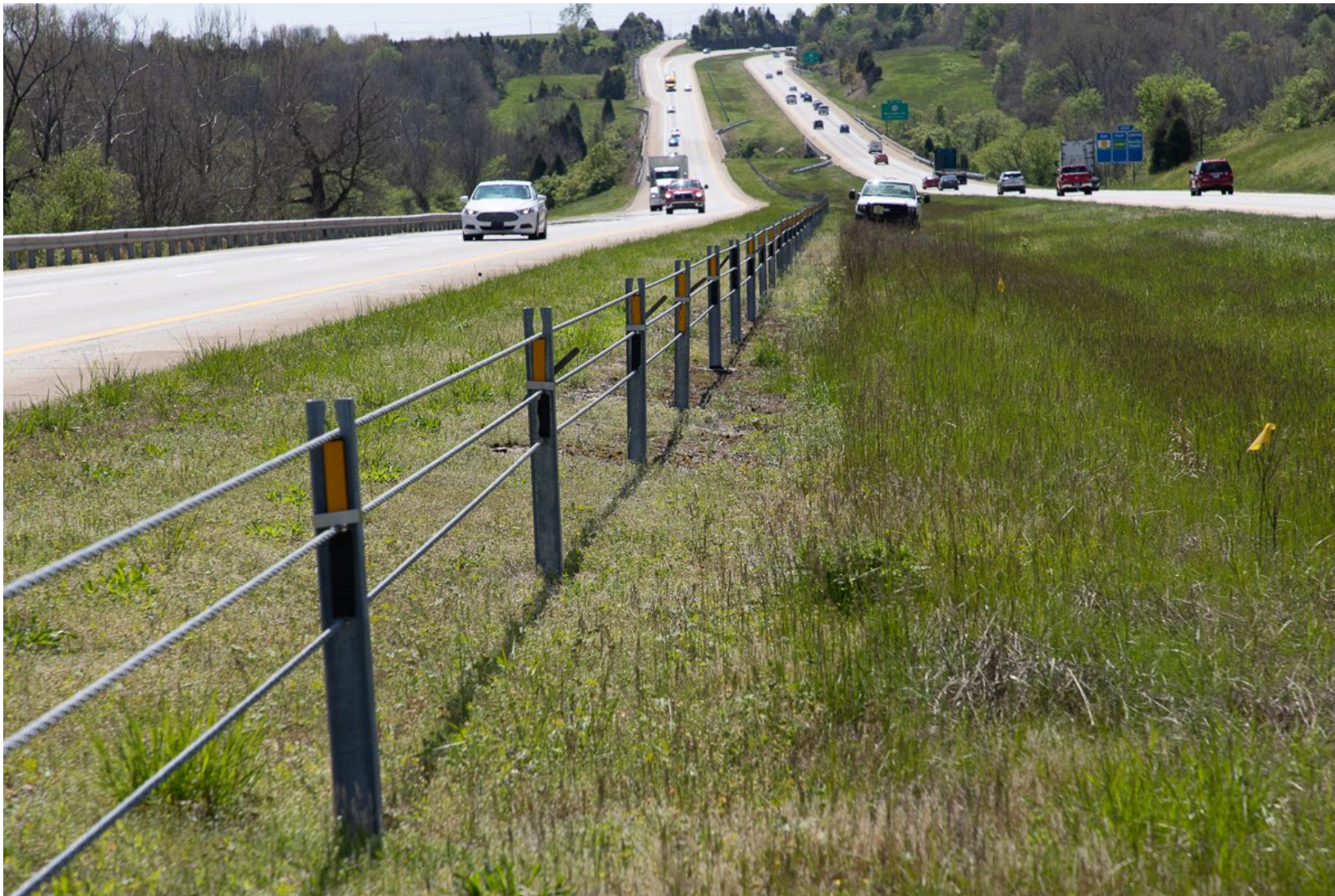
Figure 2: View of Plots in the Cable Barrier Trial on April 27, 2020 (342 Days After Treatment) Visual effects of the treatments at the beginning of the next season.
